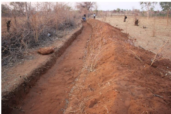
Above: Swale constructed in Tsholotsho District
