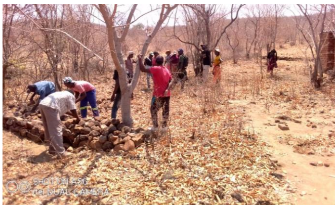
Above: Farmers making gabions in Chigwegwe gully – along Nyanyadzi River
