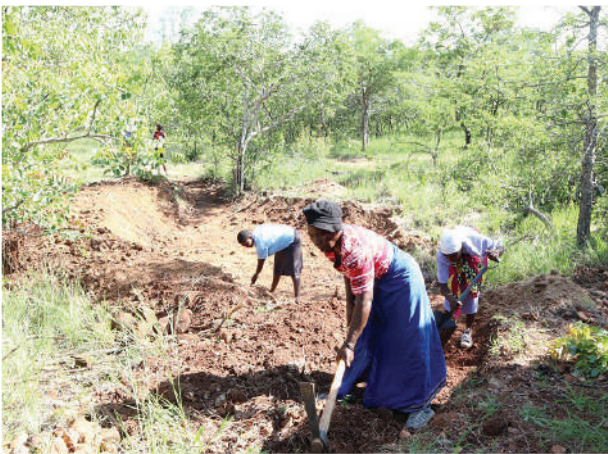
Above: Before - Preparing the dam
